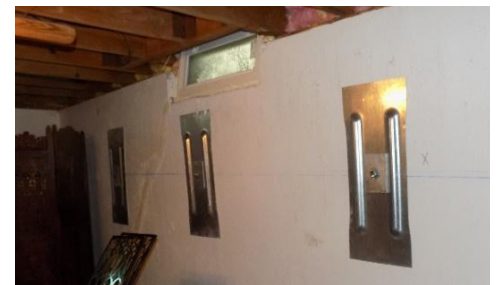
Wall Anchors to secure basement walls
